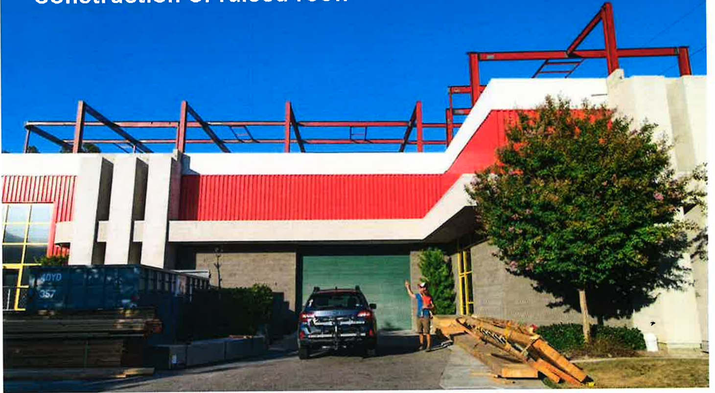
Construction of raised roof.
