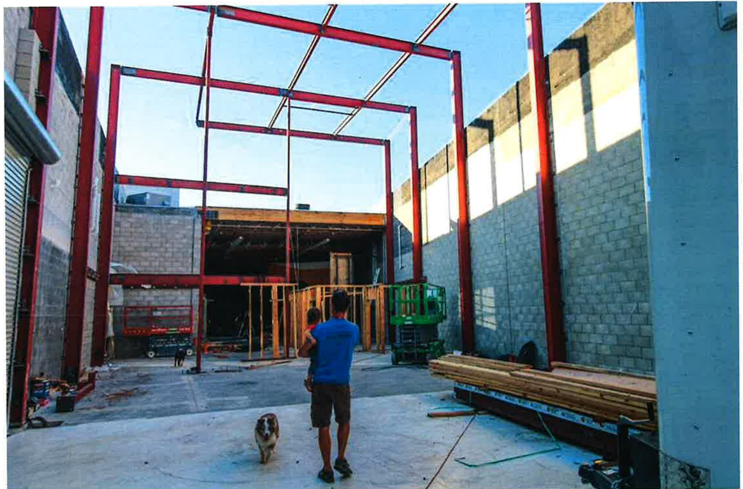
Photos - Existing Facilities
