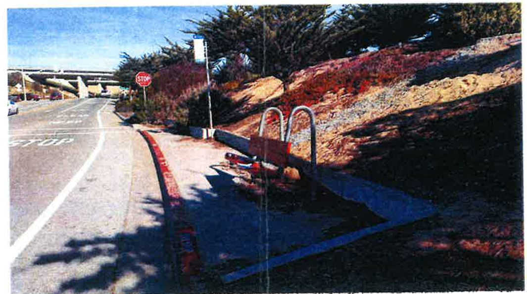
EXISTING STREET VIEW
