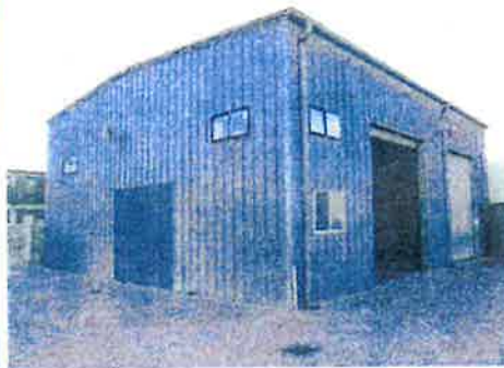
Side and Rear View
