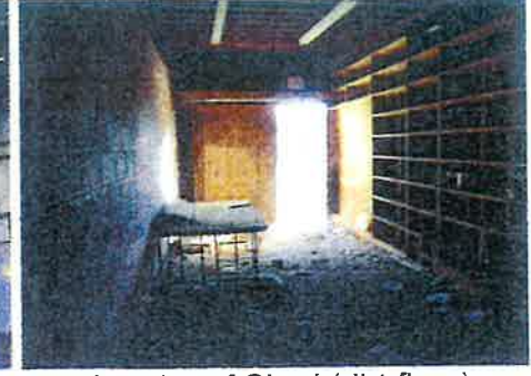
Interior of Shed (dirt floor)
