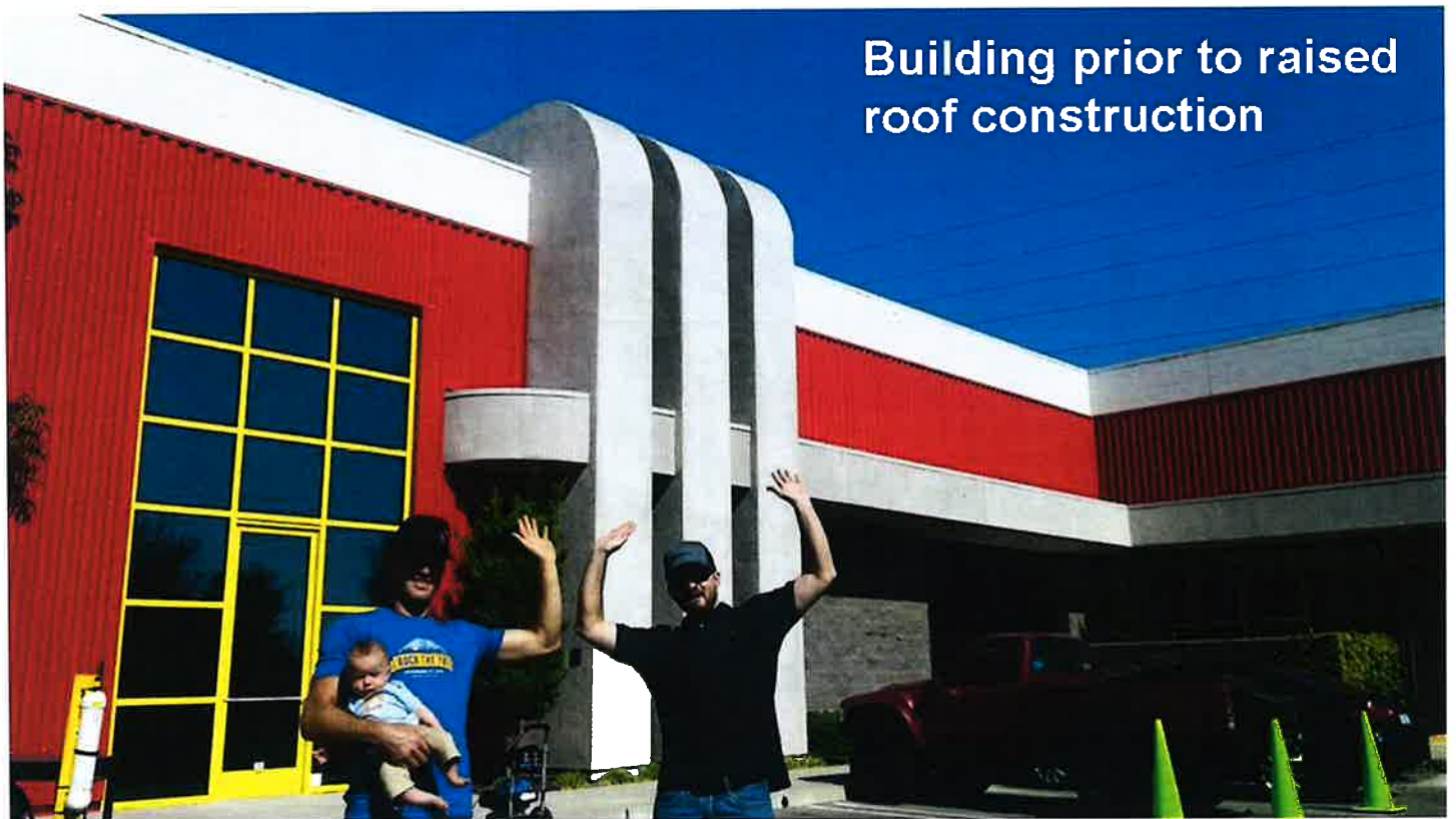
Photos - Existing Facilities
