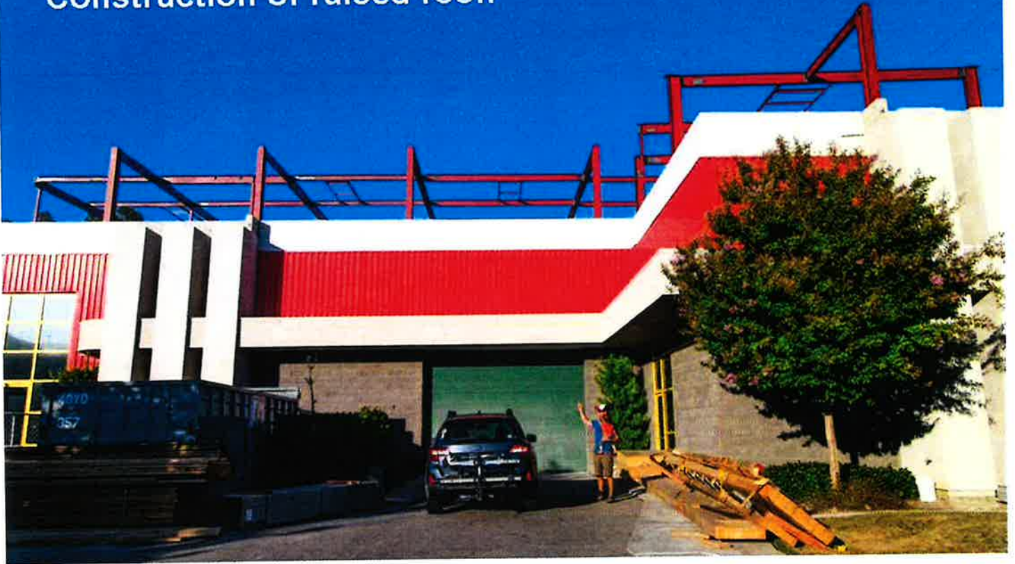
Construction of raised roof.
