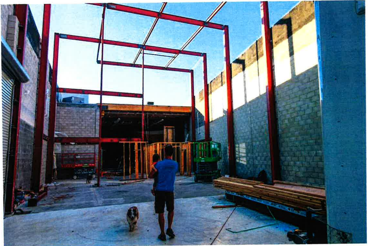
Photos - Existing Facilities
