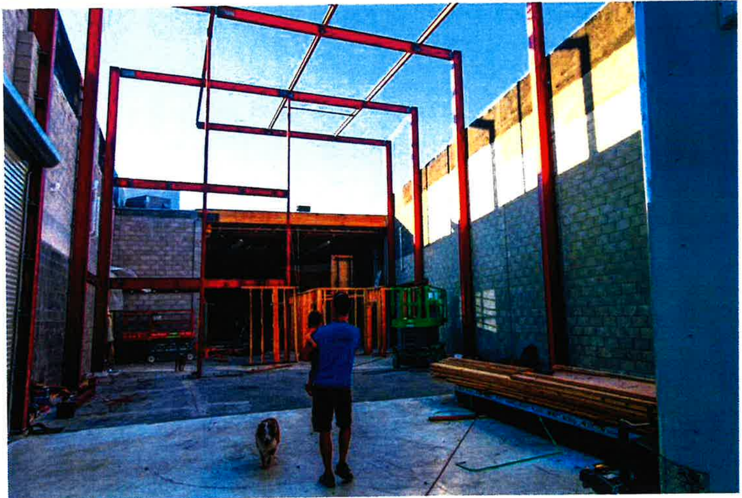
Photos - Existing Facilities
