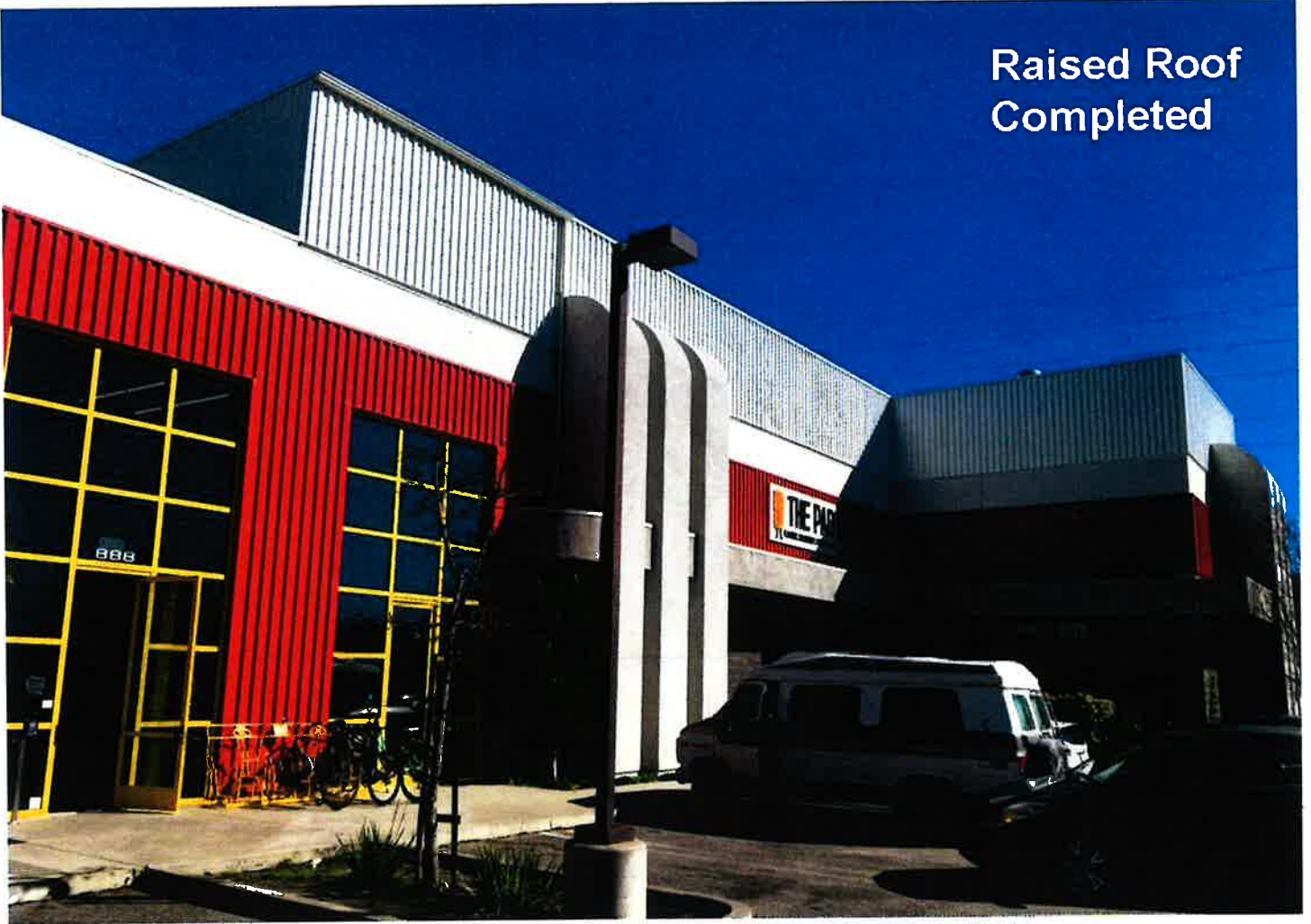
Building prior to raised roof construction
