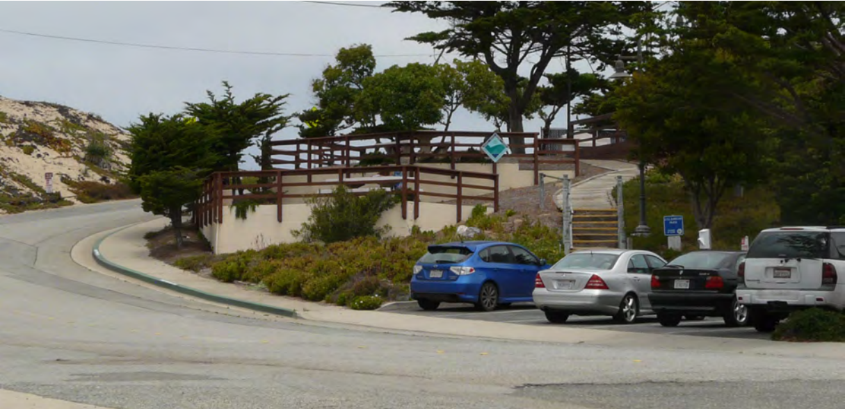
Photo F9: Pendergrass Way in front of City Hall and Calabrese Park has steep grades. Because the City owns the land in addition to the right-of-way, there is potential that an appropriate slope for wheelchairs could be accommodated here.
