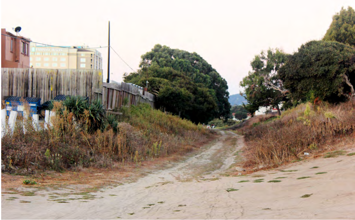
Photo A4: This section of the former Union Pacific Railroad corridor is within the City of Seaside. This view is southward from Olympia Avenue near the Seaside/Sand City limits. TAMC’s planned rapid bus/rail station location is to the left of this photograph.
