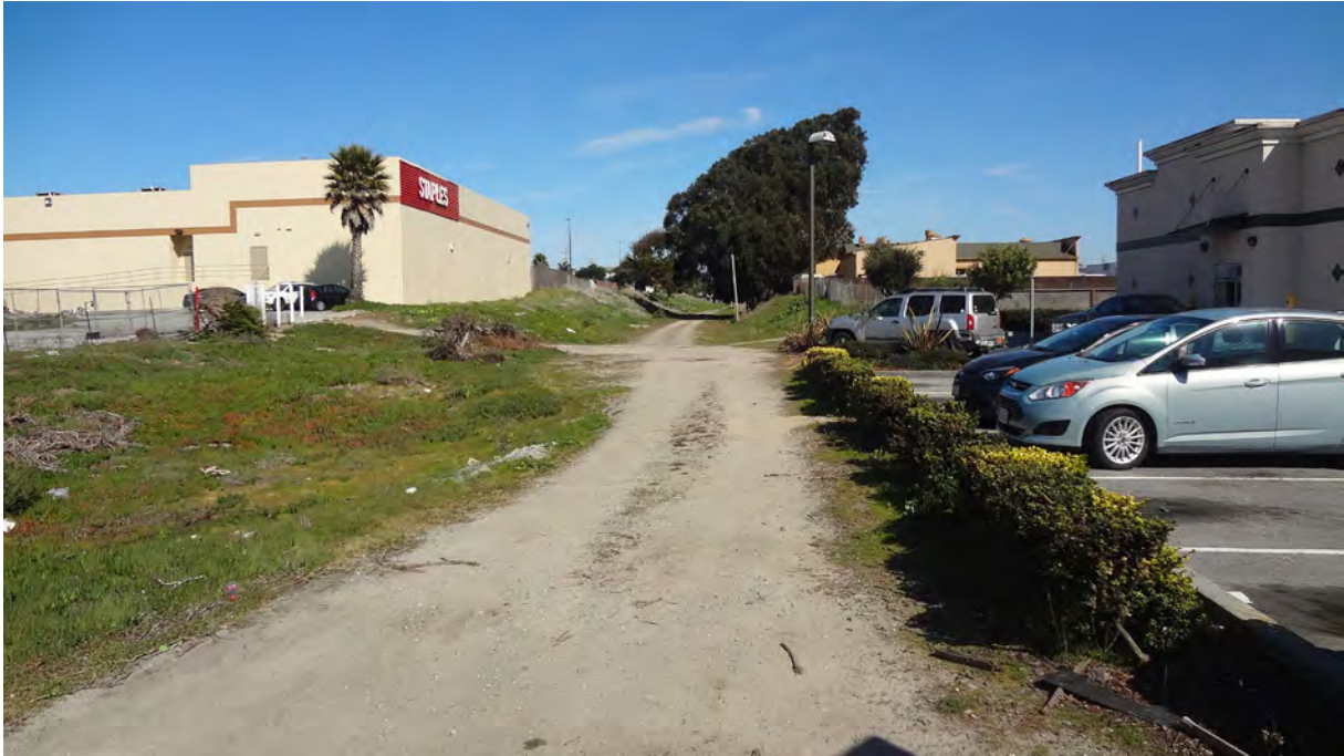
Photo A3: Former Union Pacific Railroad corridor. This segment runs from Canyon del Rey Boulevard (State Route 218) to Olympia Avenue within the City of Seaside.
