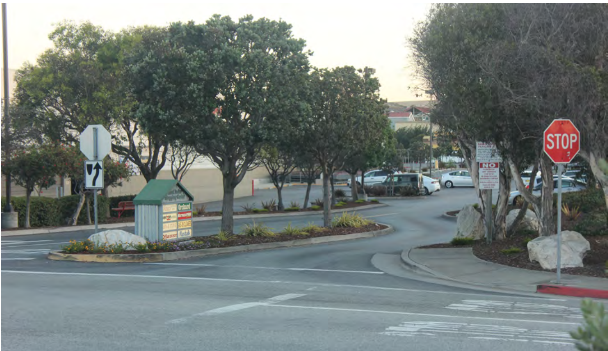
Photo E1: The entry into the Sand Dollar Shopping Center at Tioga Avenue. The sidewalks end as they curve into the entry. There is no pedestrian or wheelchair access between the corner of California Avenue and Tioga Avenue and the Costco store entrance. The only walking path is through the landscaping and the parking lot for the Costco tire center, or on the vehicle lanes.
