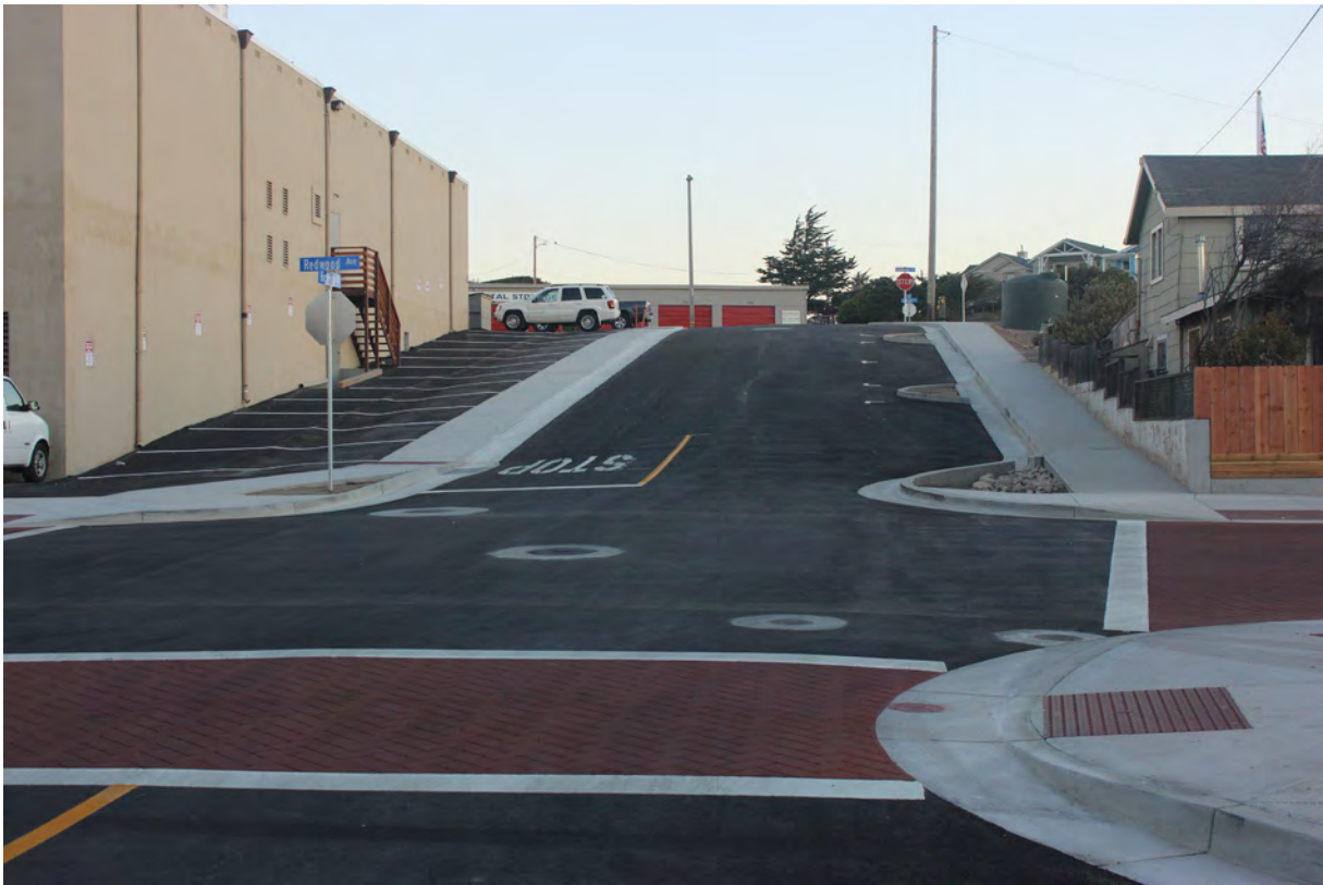
Photo F8: This photograph is taken at the Redwood Avenue and Hickory Street intersection, looking north towards the City Hall, and shows how the grade of Hickory Street is too steep for wheelchair access. This block was recently rebuilt to add sidewalks on the right side, but the grade and narrow right-of-way precluded attaining a slope suitable for wheelchairs.
