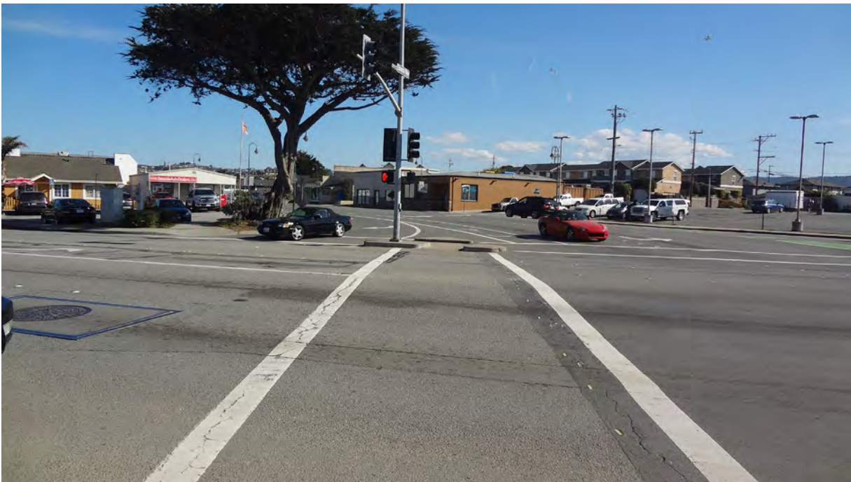
Photo A5: Pedestrian crossing of Del Monte Boulevard between Contra Costa Street and Broadway Avenue in the City of Seaside. This intersection is off-set, with Contra Costa Street about 200 feet to the left of the photo location. TAMC’s planned rapid bus/rail station location is behind this photo location.
