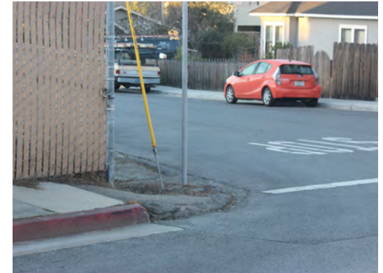
④ Sidewalk ends abruptly with obstructions.
