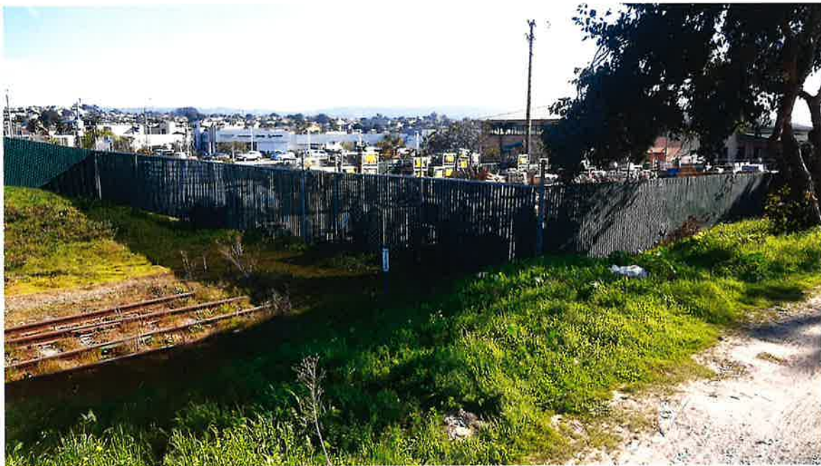
Photo D3: The tracks run through the Granite Construction yard. The company has a retail building on Del Monte Avenue in Seaside and a batch plant on California Avenue in Sand City. Granite Construction has a lease with the Transportation Agency for Monterey County for this portion of the railroad corridor that runs between its two sites.
