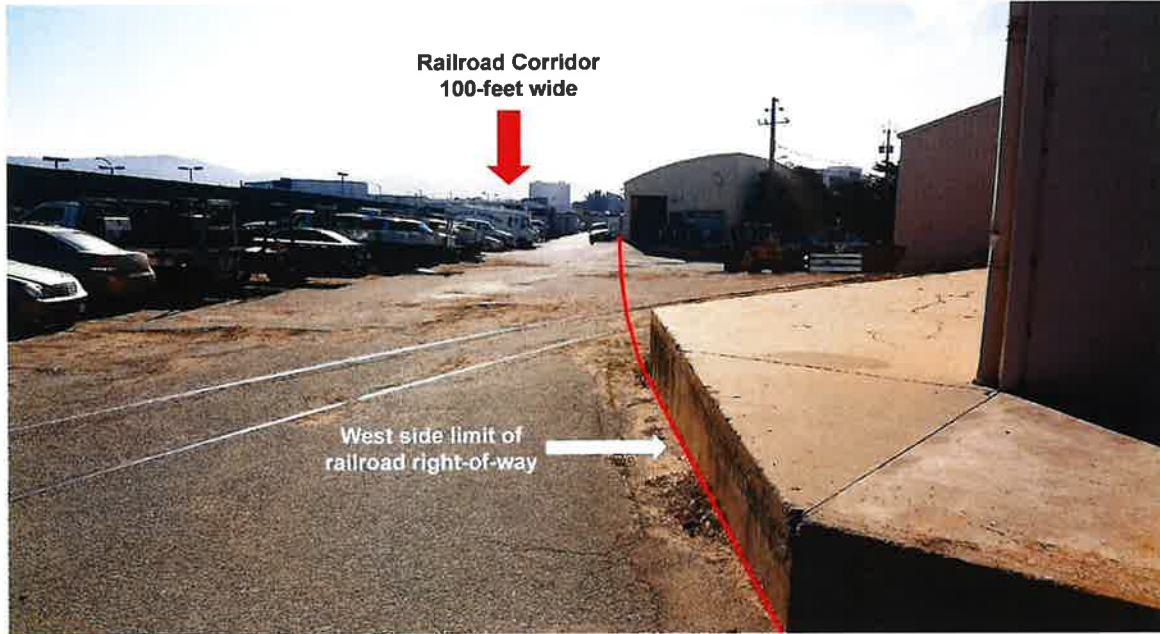
Photo D2: The railroad corridor behind a business located on Redwood Avenue. The tracks in the photograph are a siding; the main tracks continue behind the warehouse where cars are parked.
