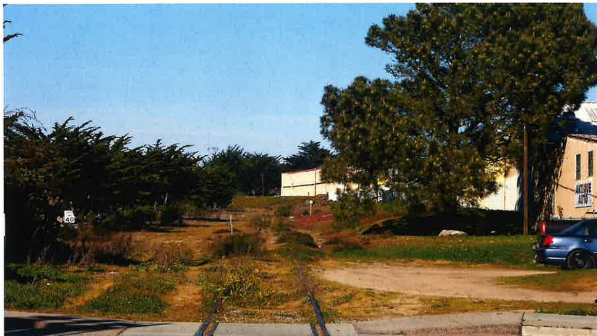
Photo D5: North of Playa Avenue the railroad corridor is empty as it runs between California Avenue in Sand City and the back of buildings located on Del Monte Boulevard in Seaside.
