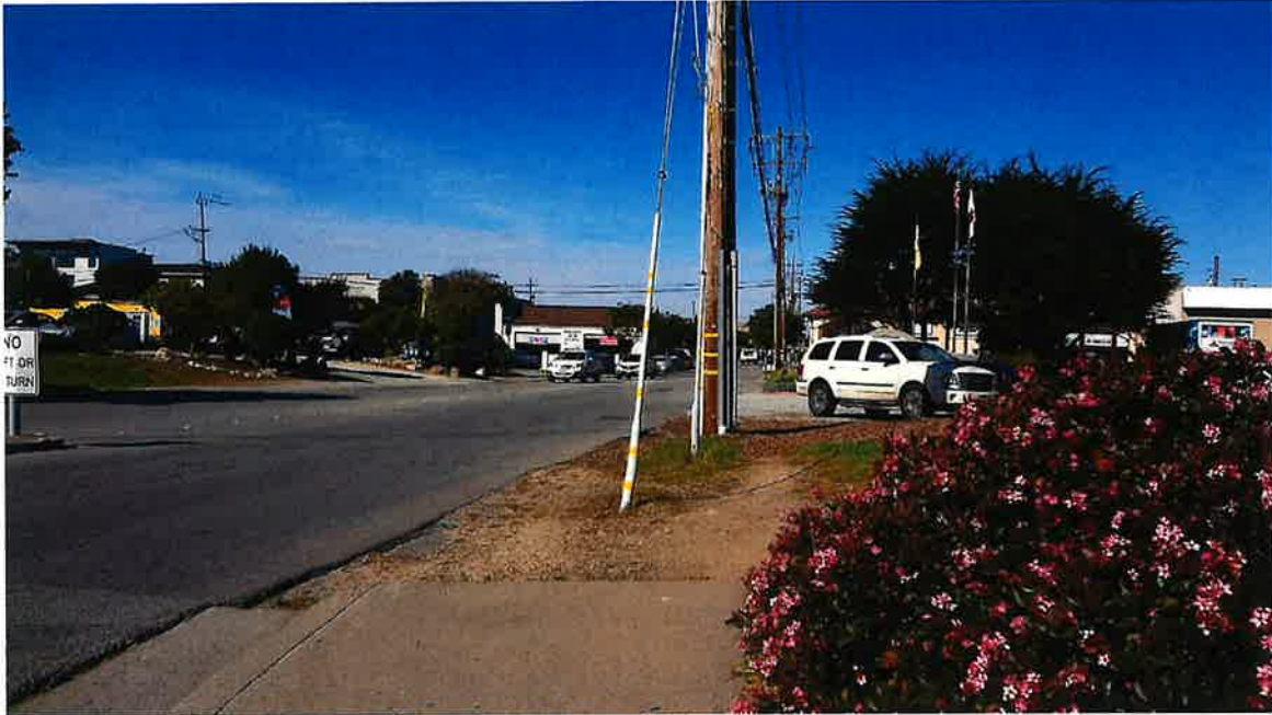
Photo F2: This photograph is taken from Contra Costa Street upon entering Sand City from Del Monte Boulevard, and shows the lack of sidewalk within the railroad corridor. Both sides of Contra Costa Street are missing sidewalks in this area.
