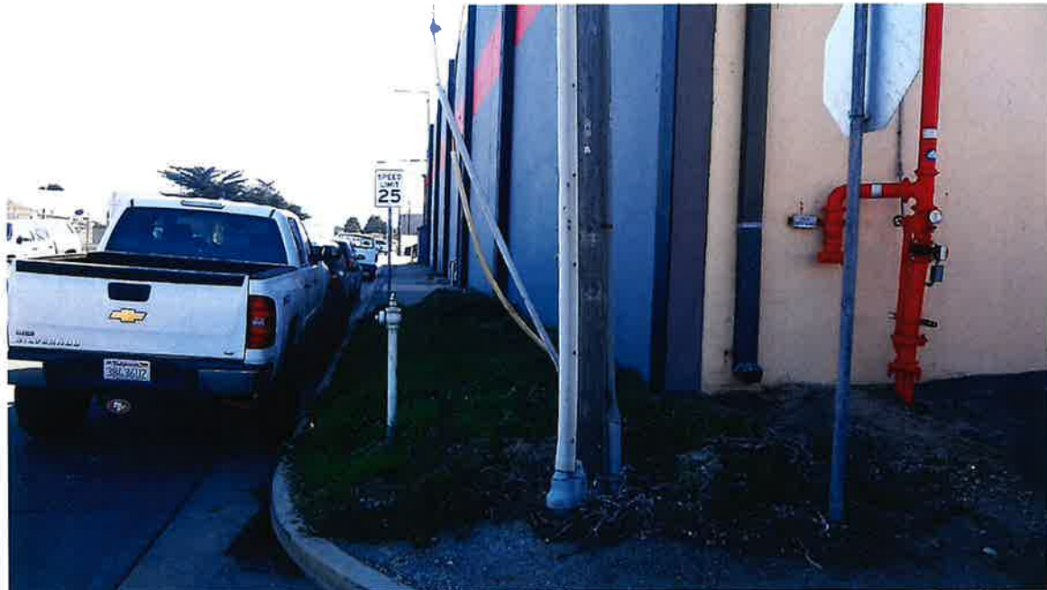
Photo F3: This photograph shows the lack of wheelchair ramps and the lack of complete sidewalks at the southeast intersection of Catalina Street and Ortiz Avenue. The City has preliminary draft public improvement plans to rectify this as part of its Stormwater Proposition 1 Grant endeavors.
