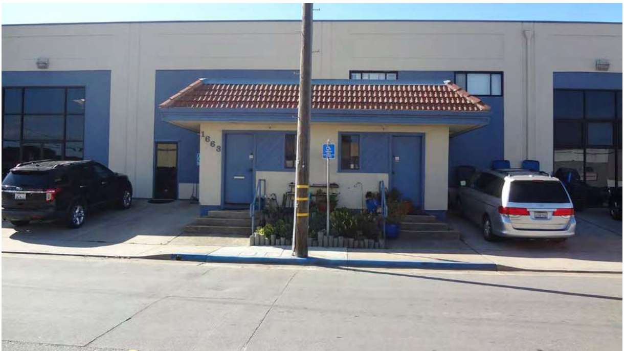
Photo F1: On-street accessible parking space on Catalina Street serving the adjacent business. There are approximately 16 accessible parking spaces in the West End District, but they may not all fully meet the requirements of the Americans with Disabilities Act.
