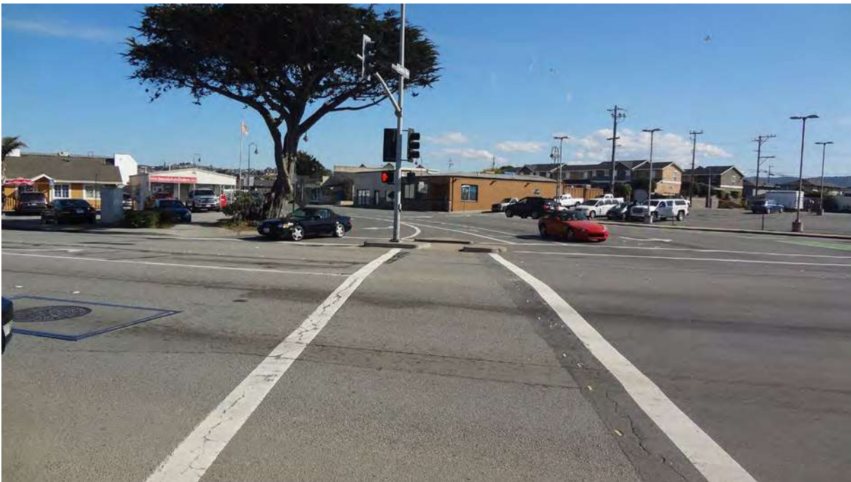
Photo A5: Pedestrian crossing of Del Monte Boulevard between Contra Costa Street and Broadway Avenue in the City of Seaside. This intersection is off-set, with Contra Costa Street about 200 feet to the left of the photo location. TAMC’s planned rapid bus/rail station location is behind this photo location.
