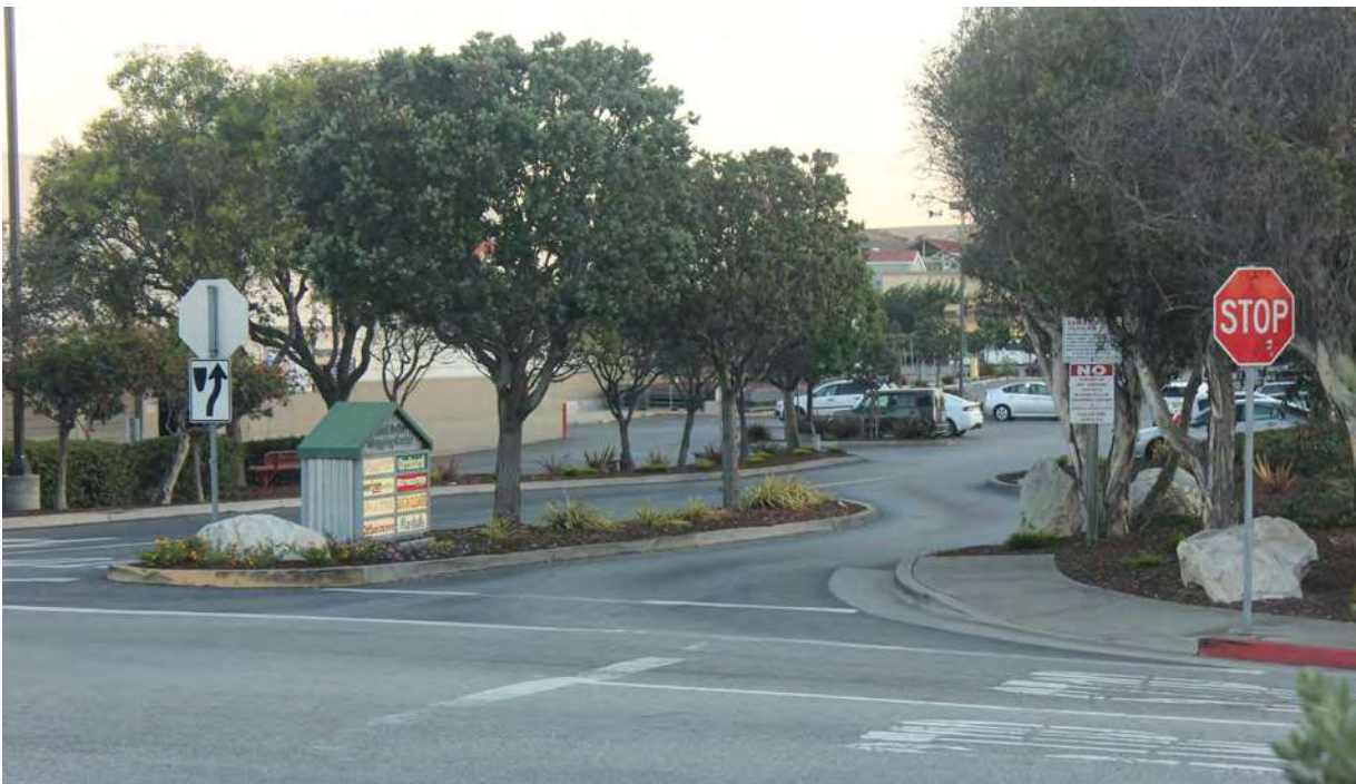
Photo E1: The entry into the Sand Dollar Shopping Center at Tioga Avenue. The sidewalks end as they curve into the entry. There is no pedestrian or wheelchair access between the corner of California Avenue and Tioga Avenue and the Costco store entrance. The only walking path is through the landscaping and the parking lot for the Costco tire center, or on the vehicle lanes.
