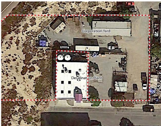
Public Works Yard / Desalination Plant
