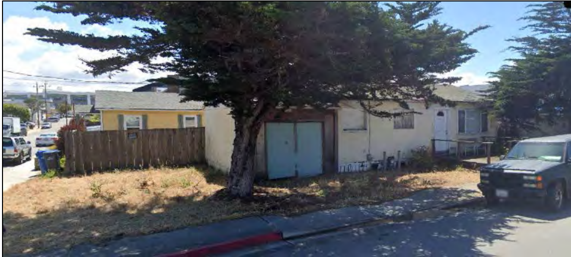
Figure C-12 1712 Catalina Street, Site #5
