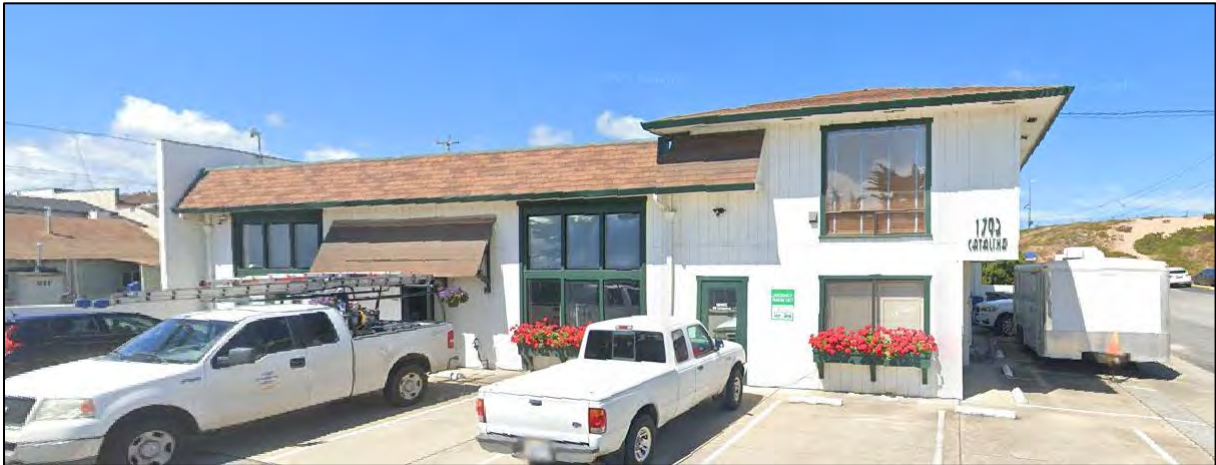
Figure C-11 1793 Catalina Street, Site #4
