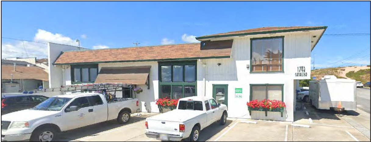
Figure C-11 1793 Catalina Street, Site #4
