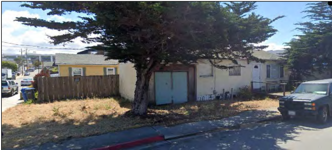
Figure C-12 1712 Catalina Street, Site #5
