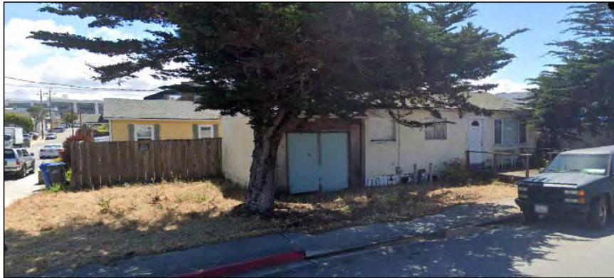
Figure C-14 1712 Catalina Street, site #7
