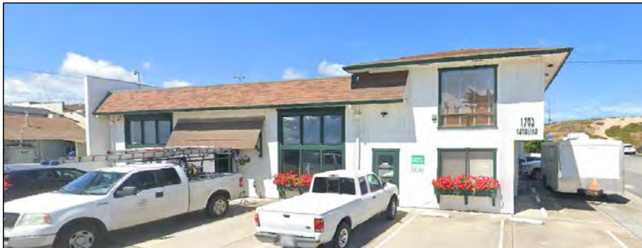
Figure C-11 1793 Catalina Street, Site #4
