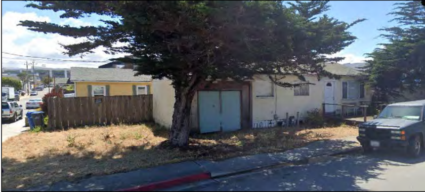
Figure C-12 1712 Catalina Street, Site #5
