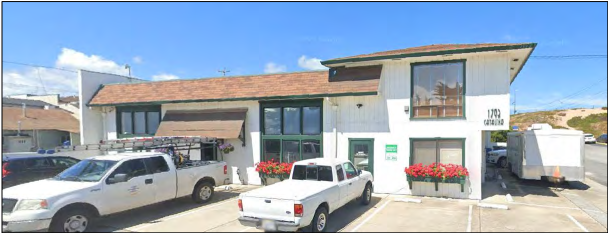
Figure C-11 1793 Catalina Street, Site #4
