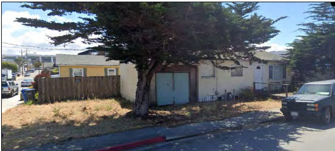
Figure C-12 1712 Catalina Street, Site #5
