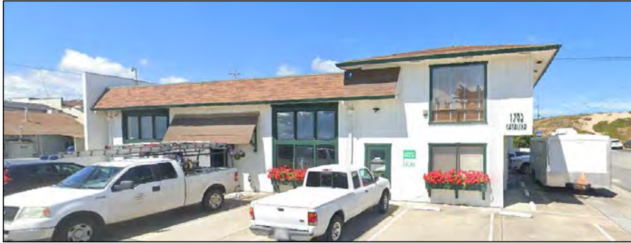
Figure C-13 1793 Catalina Street, site #6
