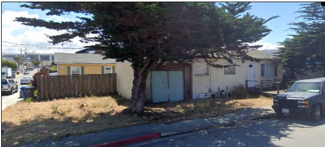
Figure C-12 1712 Catalina Street, Site #5
