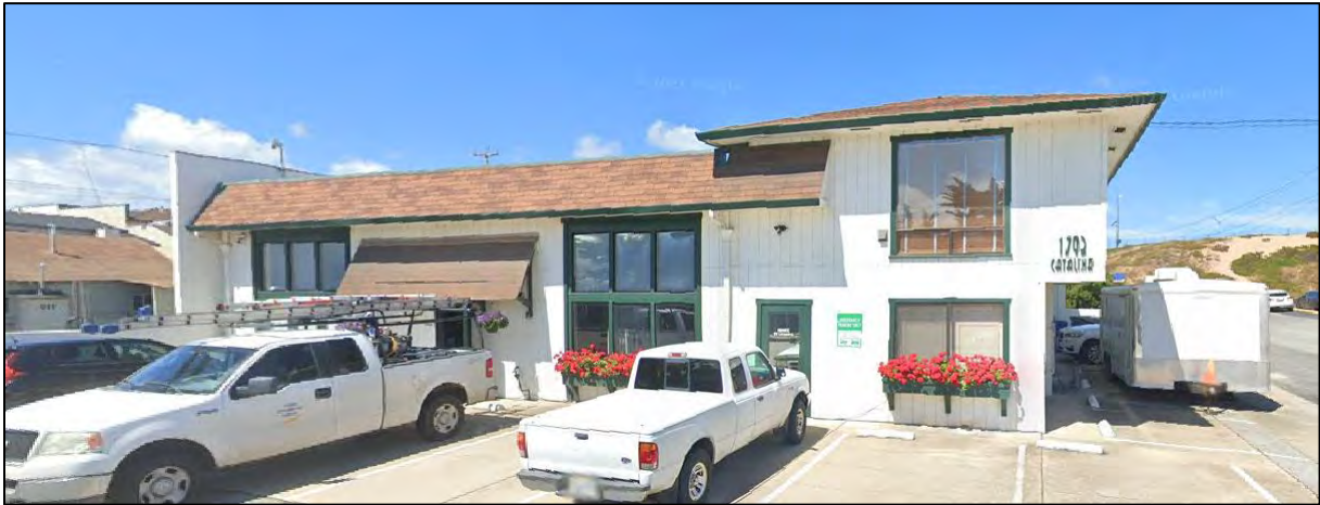
Figure C-11 1793 Catalina Street, Site #4
