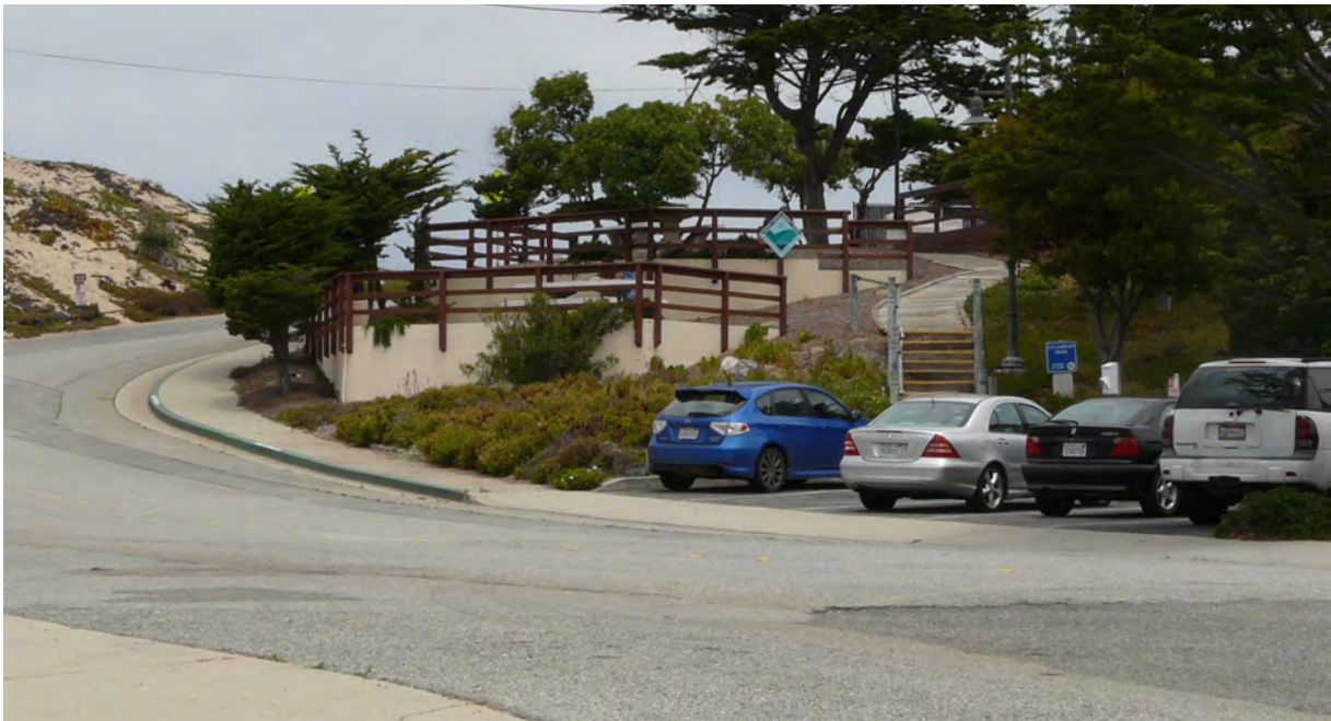
Photo F9: Pendergrass Way in front of City Hall and Calabrese Park has steep grades. Because the City owns the land in addition to the right-of-way, there is potential that an appropriate slope for wheelchairs could be accommodated here.
