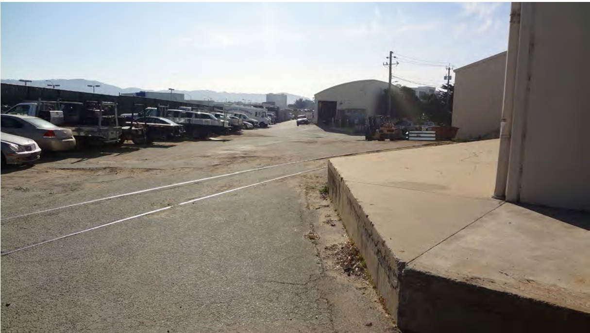
Photo D2: The railroad corridor behind a business located on Redwood Avenue. The tracks in the photograph are a siding; the main tracks continue behind the warehouse where cars are parked.
