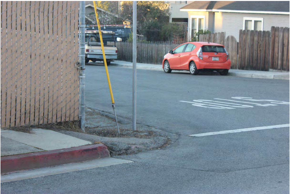
Photo F12: This photograph is taken on California Street just north of City Hall, where there is a sidewalk on one side of the street frequently blocked by parked vehicles, and no sidewalk on the other side.
