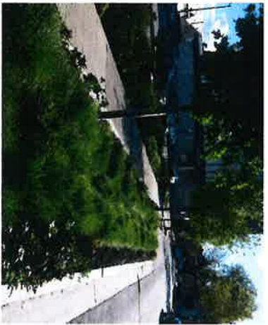
Stormwater Curb Extension
