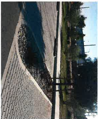
Head-in Parking Permeous Paving
