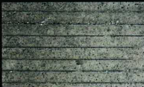
BOARD – FORMED WEATHERED CONCRETE CLADDING
