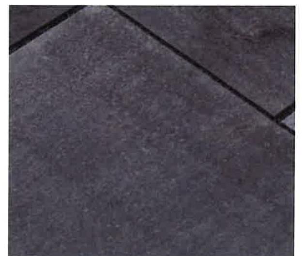
SAW CUT SANDSTONE PAVERS
